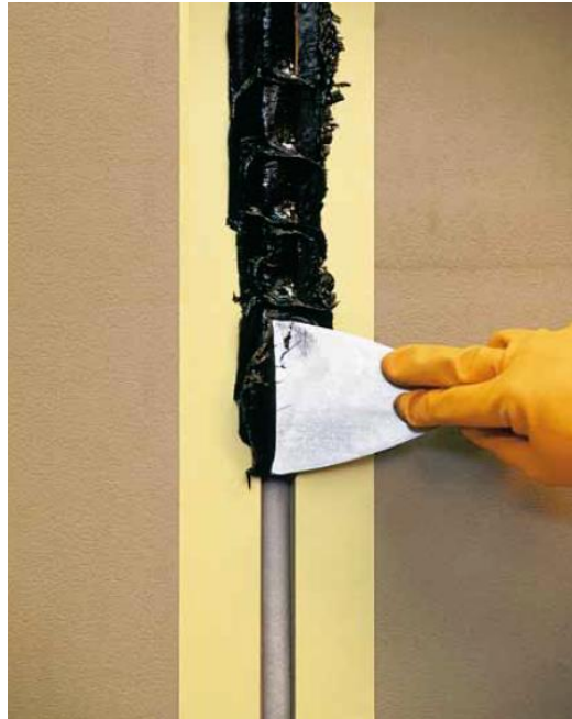
Application verticale de l'Esotrope Pub HR 25 thixotrope
